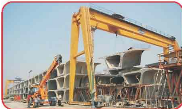
Wadala Segment Manufacturing Plant (Mumbai)
