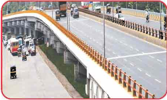
Dindoshi Flyover (Mumbai)
