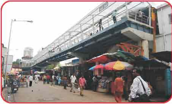
Grant Road Skywalk (Mumbai)
